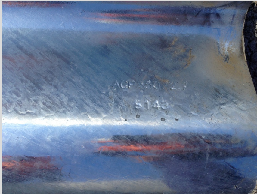
Typical view of the hard stamped details on the guardrail panel
